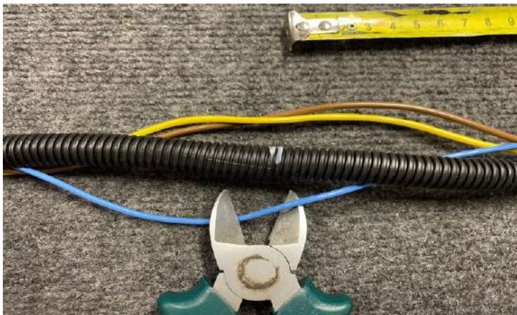
Pull out the wires in the marked place. Snack on the blue wire.
